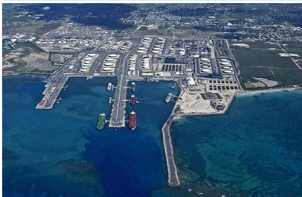
View of Current HOVENSA Facility
