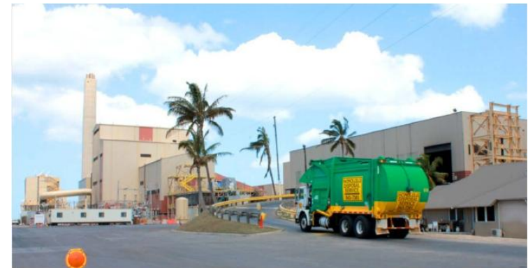
Figure 2: 50 MW Waste-to-Energy Facility in Oahu, Hawaii
