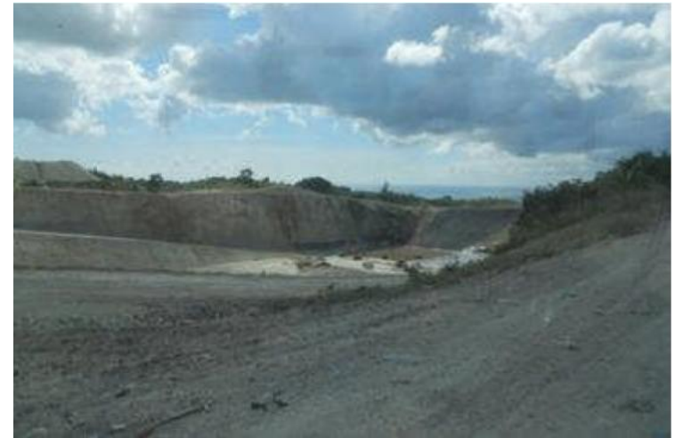
Future site for Mangrove Pond Green Energy Complex in Bridgetown, Barbados
