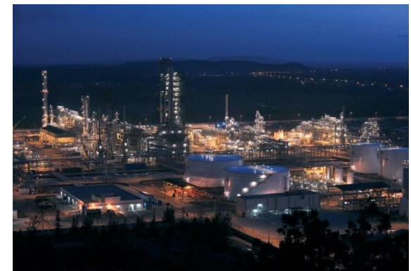
Saudi Aramco Total Refining Co (Satorp) refinery in Jubail, Saudi Arabia
