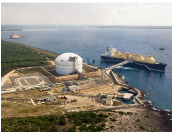
AES Corporation's LNG Import Terminal in the Dominican Republic.
